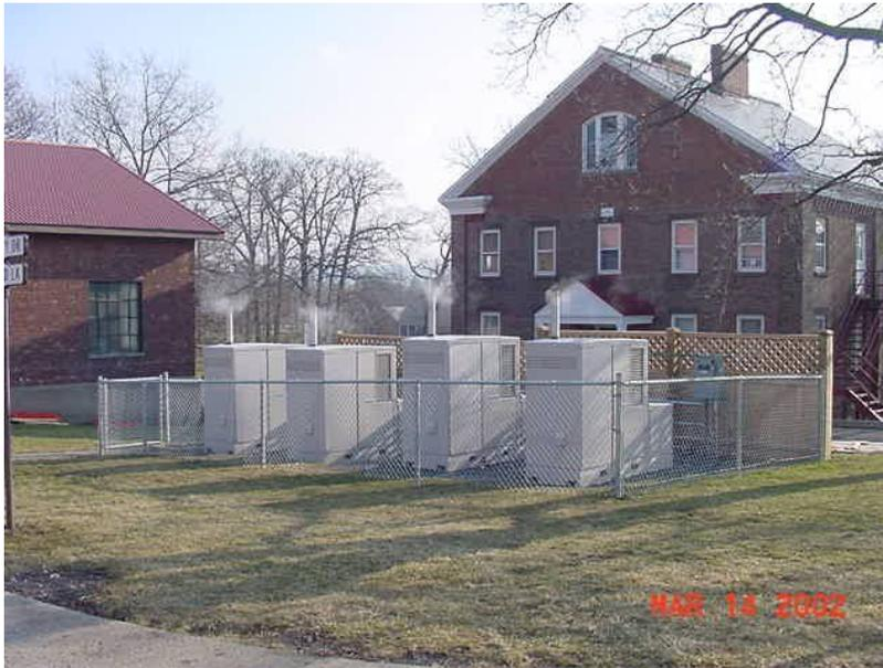
**Figure A12. Four Plug Power units installed at Watervliet Arsenal, NY.**
