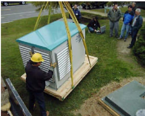
**Figure A11. Installing fuel cell at Patuxent River.**
