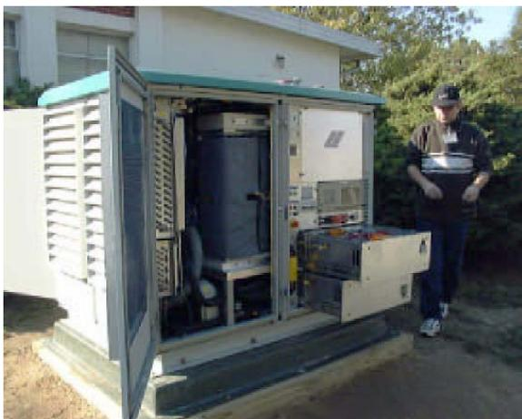
**Figure A10. Interior of H Power fuel cell.**
