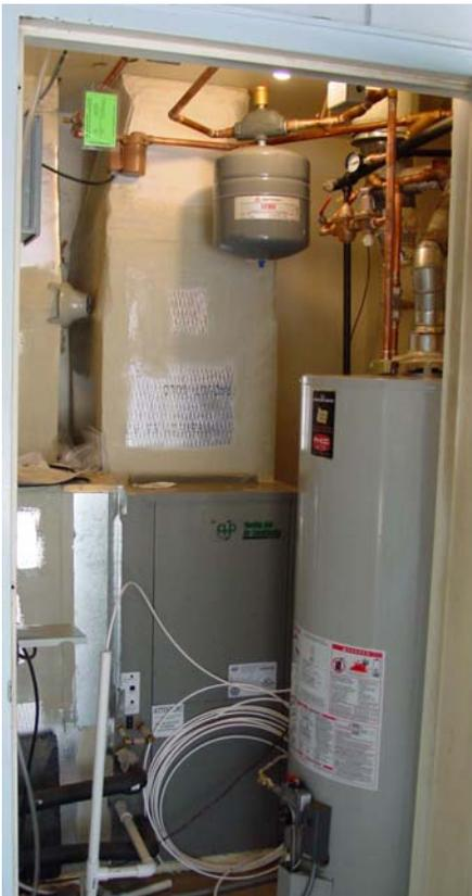
Figure A6. Thermal recovery system.
