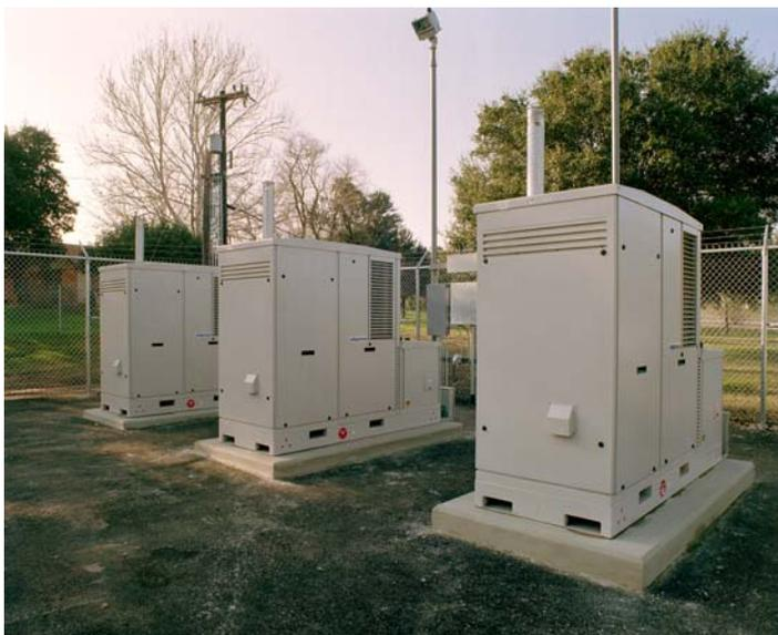
**Figure A3. Fuel cells at Brooks AFB residence.**
