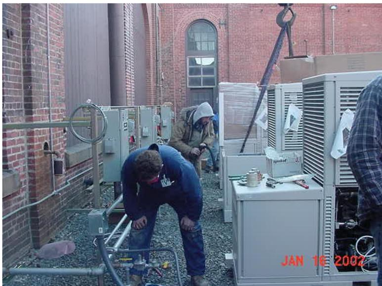
**Figure A13. Installation of PEM fuel cells at Watervliet Arsenal, NY.**
