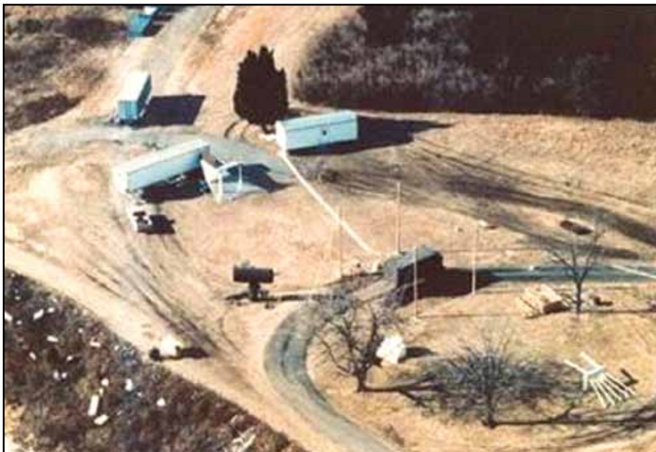
Figure 4. Transportable Oscillating Pulser System (TOPS)
