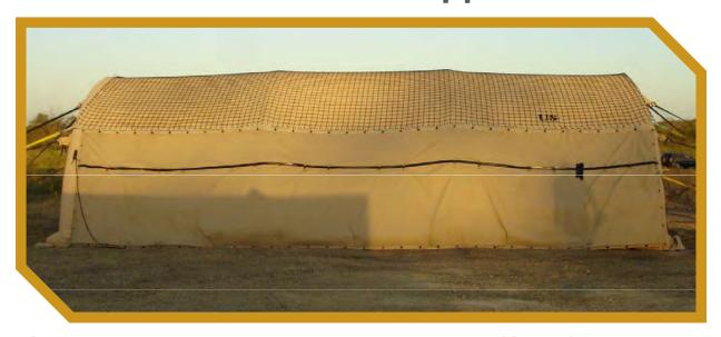
Through the Small Business Innovative Research (SBIR) program, a flexible ballistic solution was sought for an approach to protect shelters with unique arc shapes of non-traditional frame shelters.
