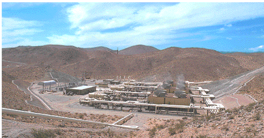
Figure E-3. Geothermal Plant at China Lake
