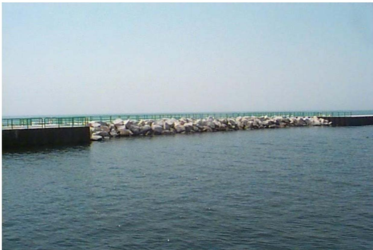
Figure 1. Pocket wave absorber at Pentwater, MI
