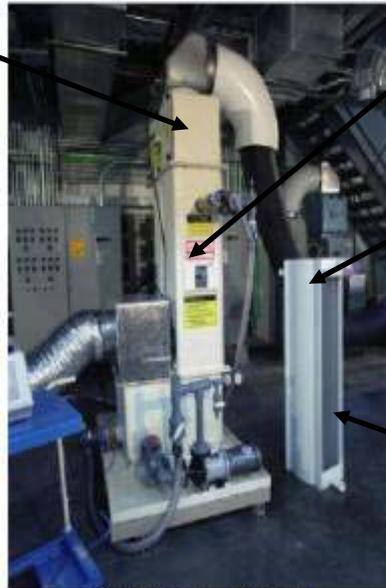
Current Conditioner: 1500 cfm, 50 gallons lithium chloride liquid desiccant "air washer"
