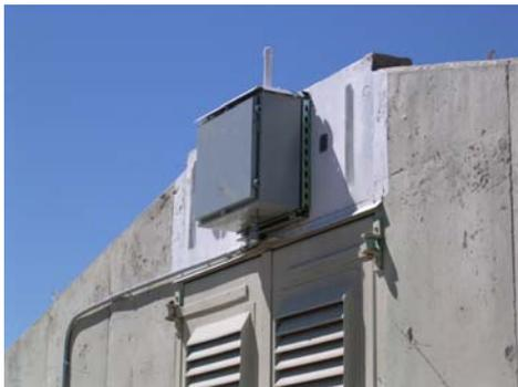
Figure 8. The PAS Store Forward Computer & RFID Tag Reader
